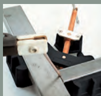
WELDING 'T' JOINTS ON SQUARE TUBE
